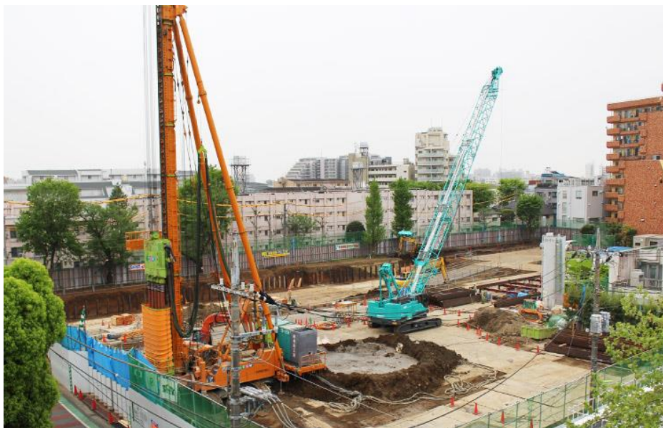
Construction underway at the New TUJ Campus in Setagaya-ku
