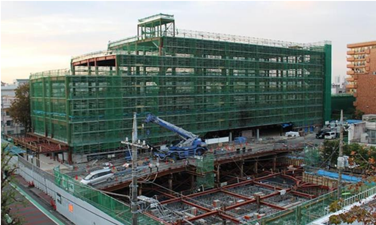
Construction is on schedule and underway at the New TUJ Campus.
